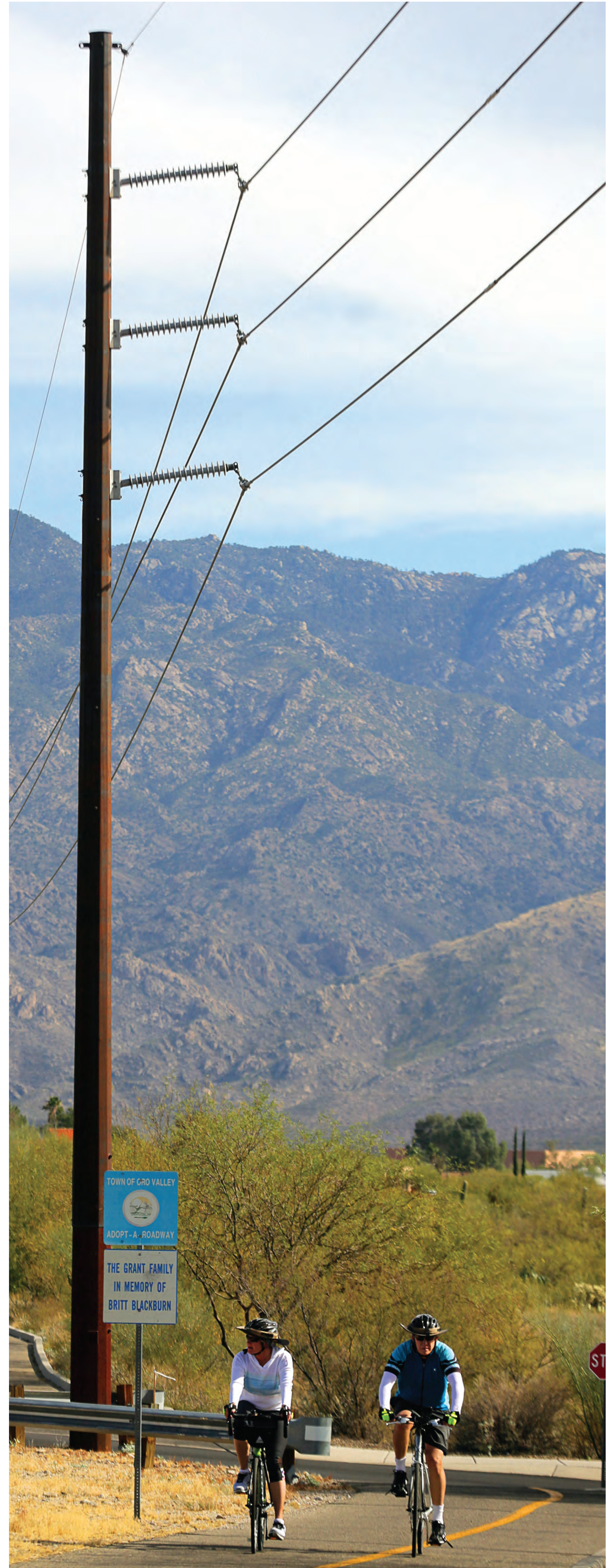
A typical weathering steel monopole supporting a 138 kilovolt transmission line
