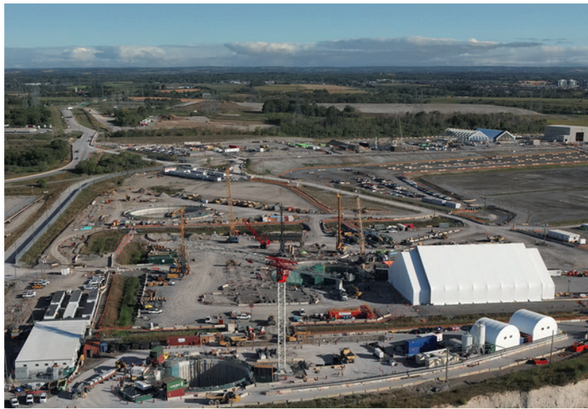
Figure 7 - Construction of GE Hitachi's BWRX-300 SMR. 11
