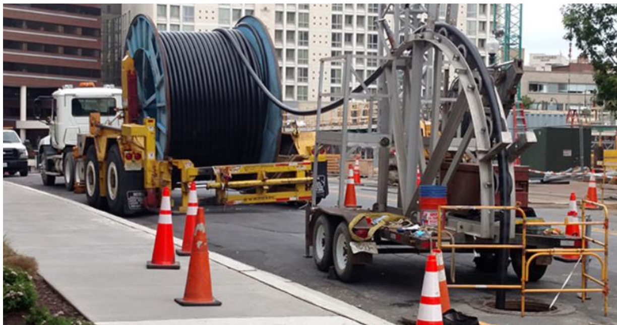
Figure 2-9 – XLPE Cable Installation
