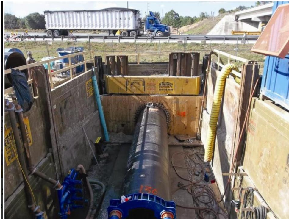
Figure 2-4 — Jack and Bore – Send Pit
