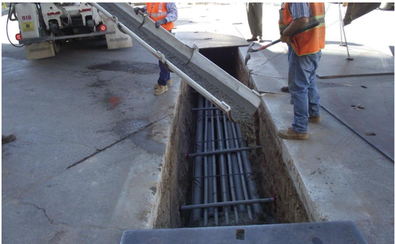
Figure 2-3— Open Trench Concrete
