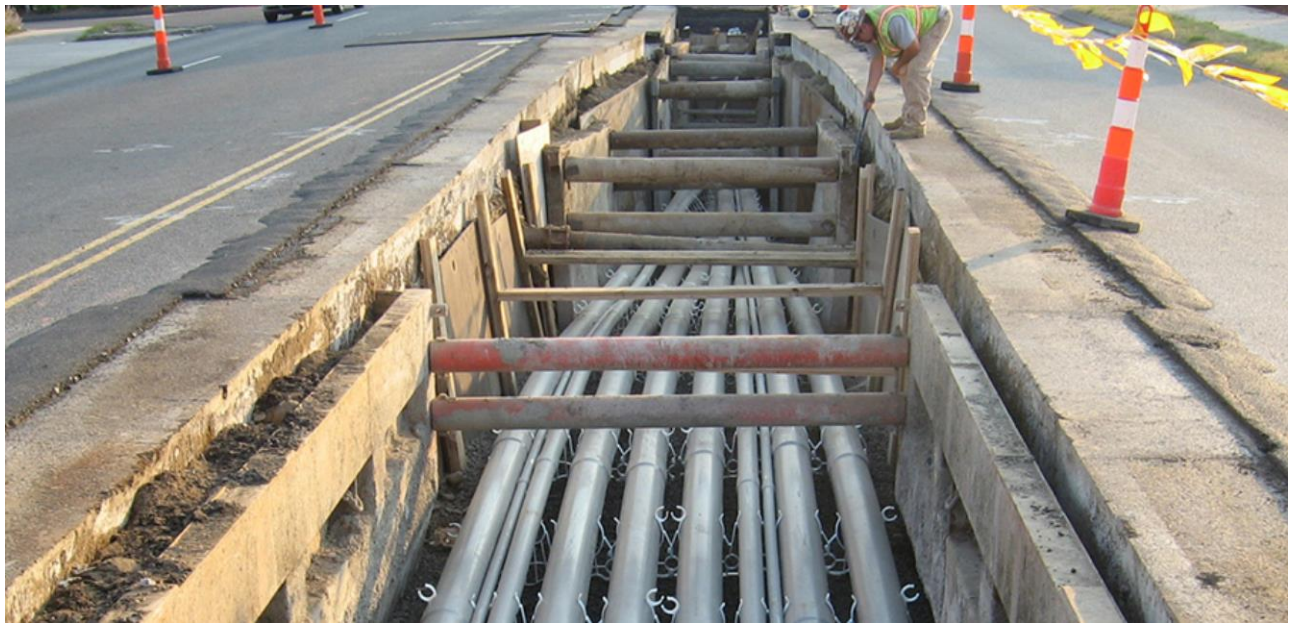
Figure 2-3— Open Trench Concrete
