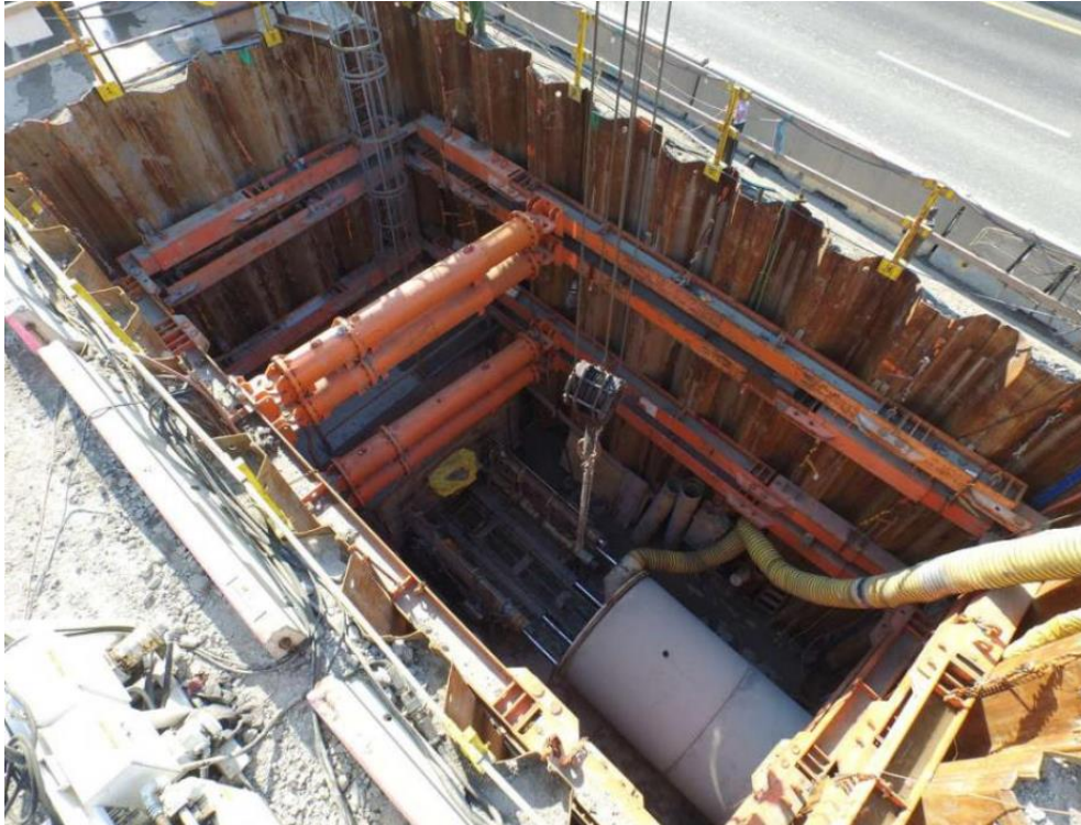
Figure 2-5 — Jack and Bore – Equipment
