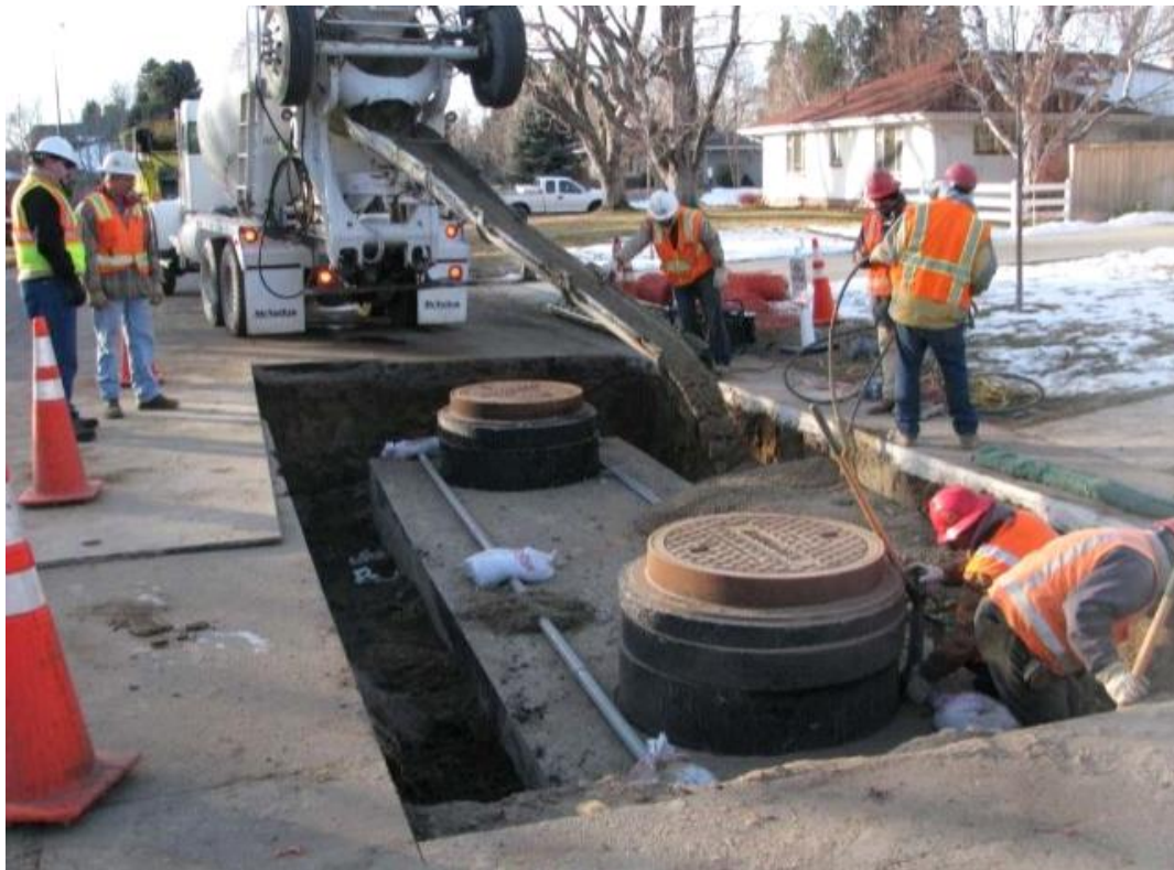
Figure 2-7 – Man Vault Backfill
