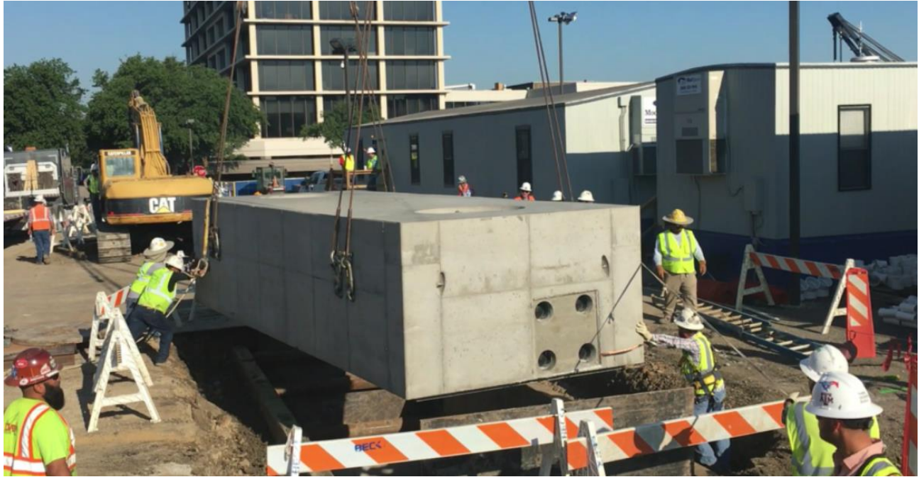
Figure 2-7 – Man Vault Backfill
