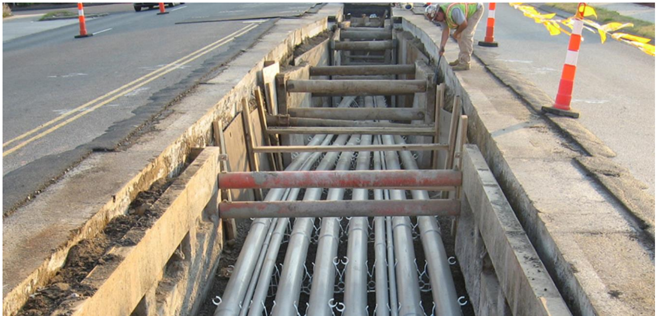
Figure 2-3— Open Trench Concrete
