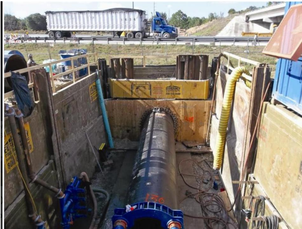
Figure 2-4 — Jack and Bore – Send Pit
