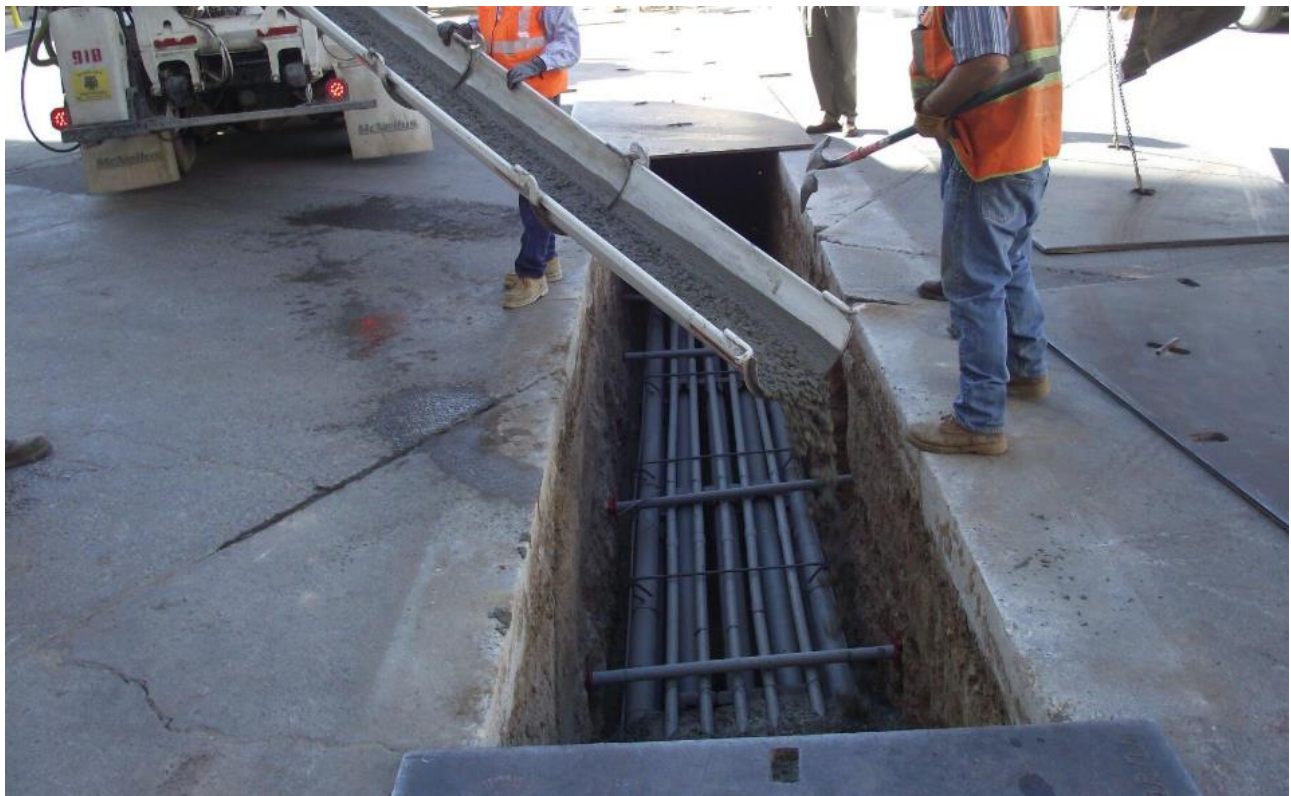
Figure 2-3— Open Trench Concrete
