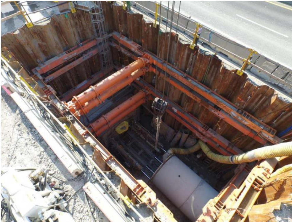
Figure 2-5 — Jack and Bore – Equipment
