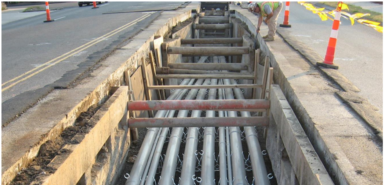
Figure 2-3— Open Trench Concrete
