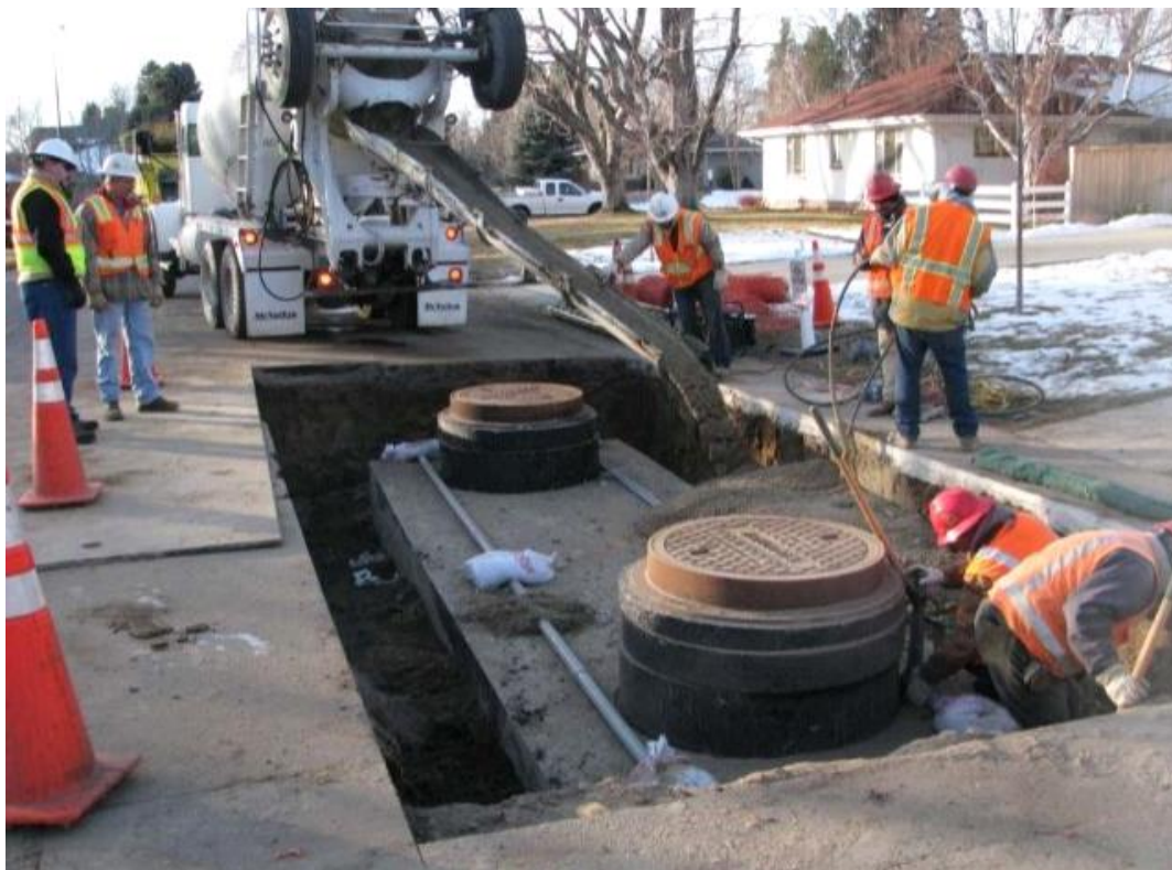
Figure 2-7 – Man Vault Backfill
