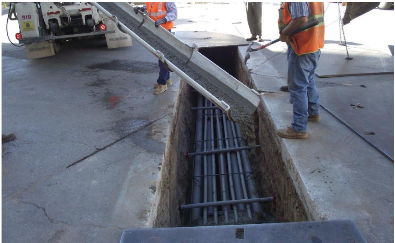
Figure 2-3— Open Trench Concrete
