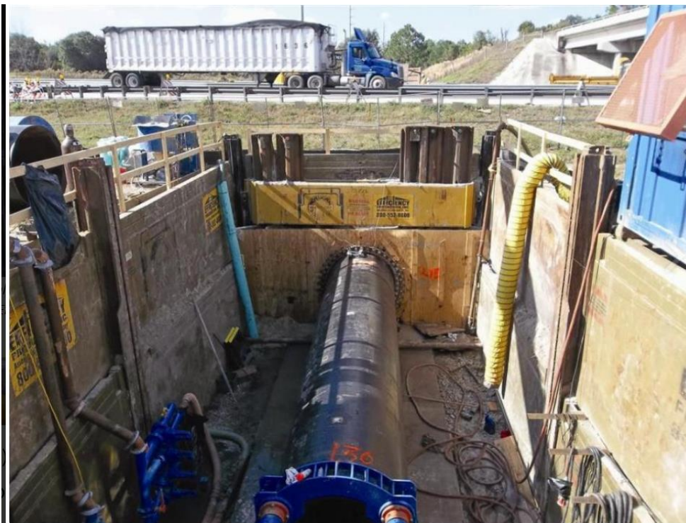
Figure 2-4 — Jack and Bore – Send Pit
