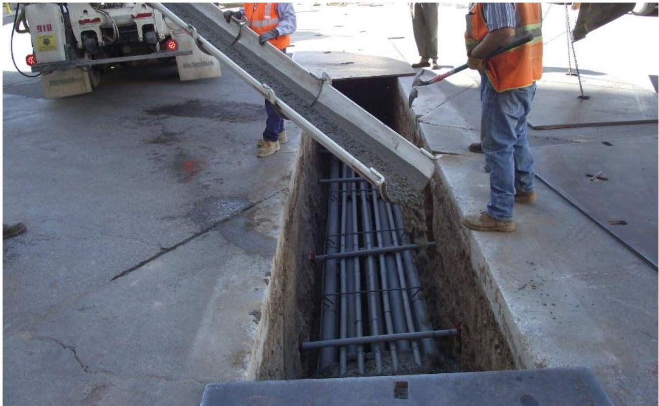
Figure 2-3— Open Trench Concrete
