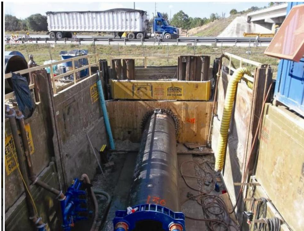
Figure 2-4 — Jack and Bore – Send Pit
