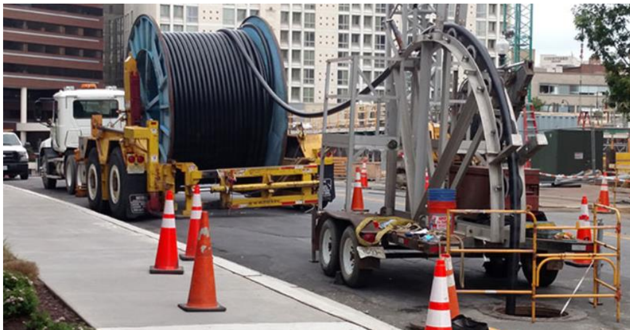
Figure 2-9 – XLPE Cable Installation
