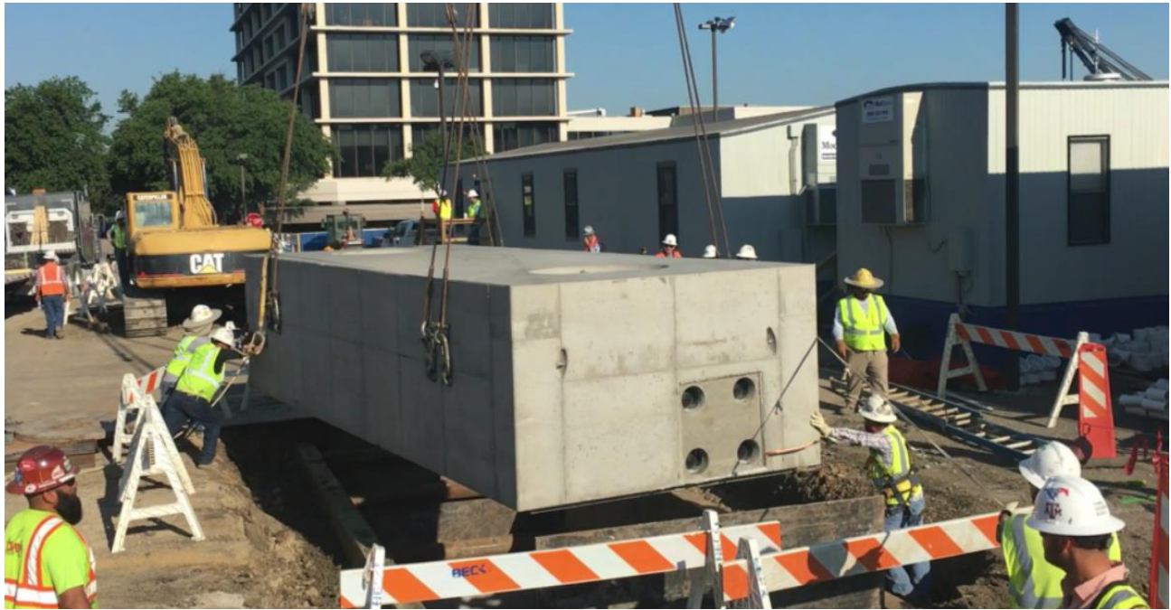
Figure 2-7 – Man Vault Backfill
