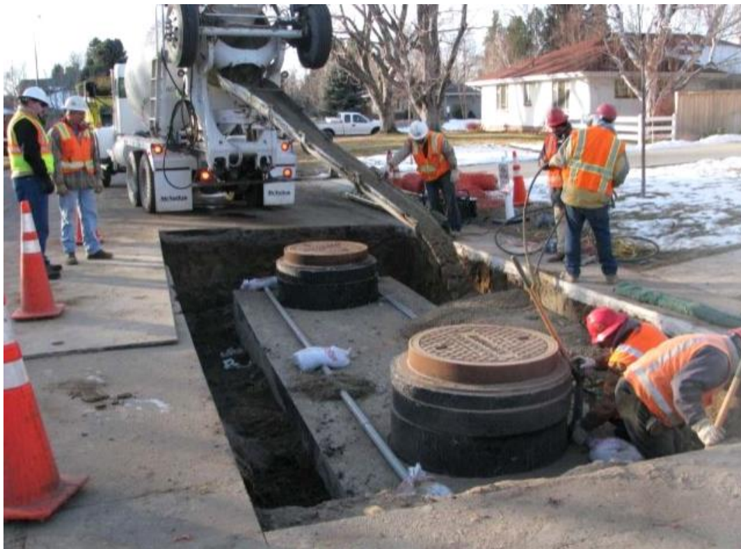
Figure 2-7 – Man Vault Backfill
