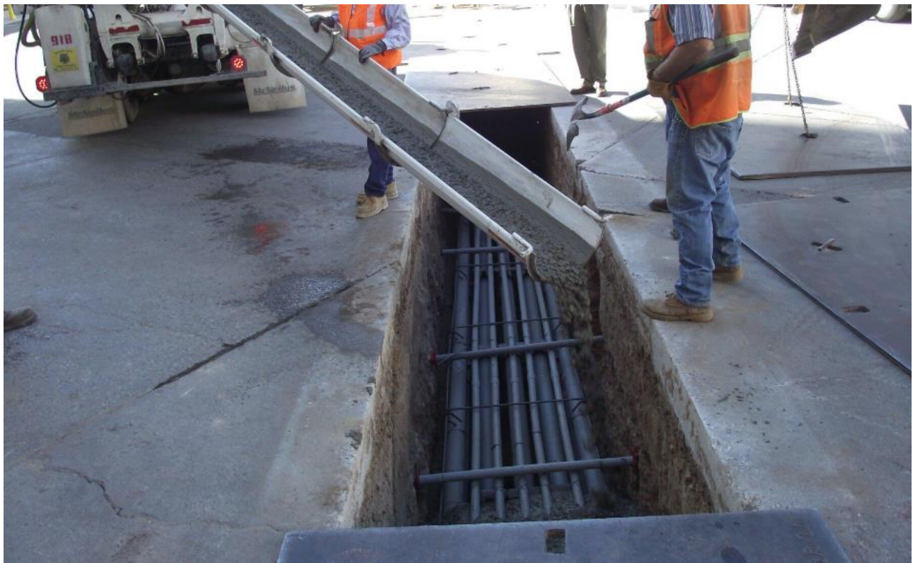
Figure 2-3— Open Trench Concrete
