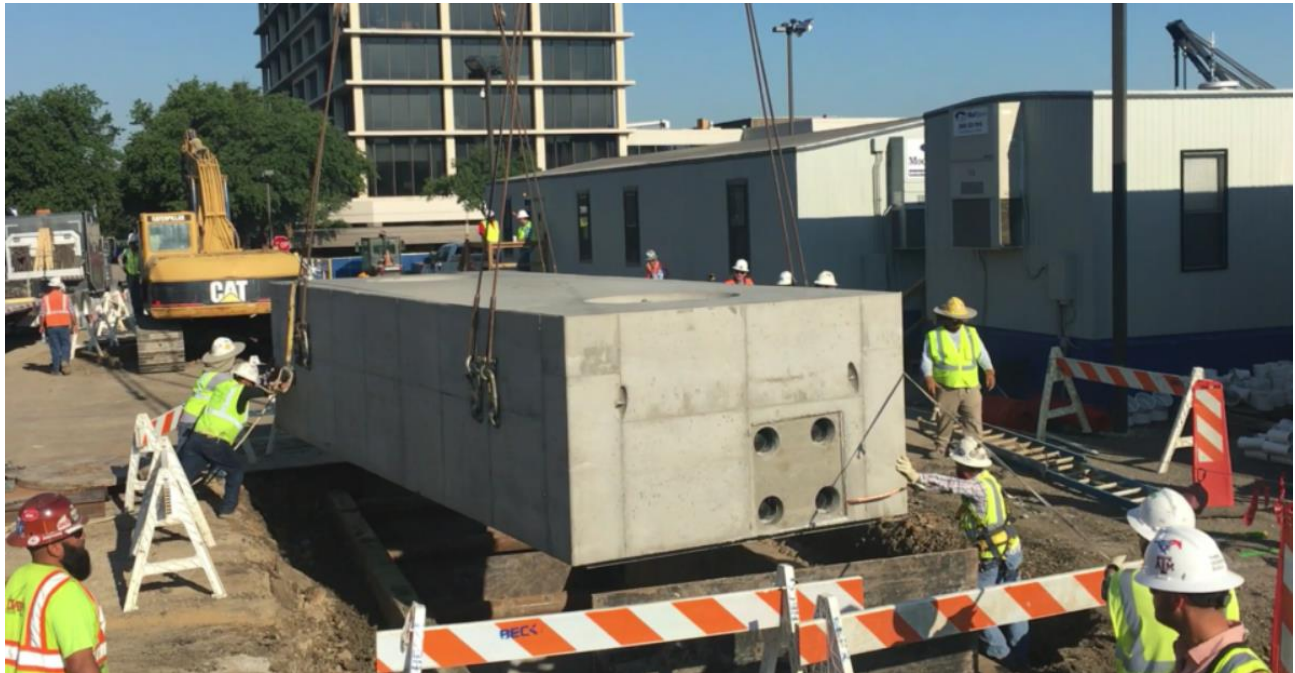
Figure 2-7 – Man Vault Backfill
