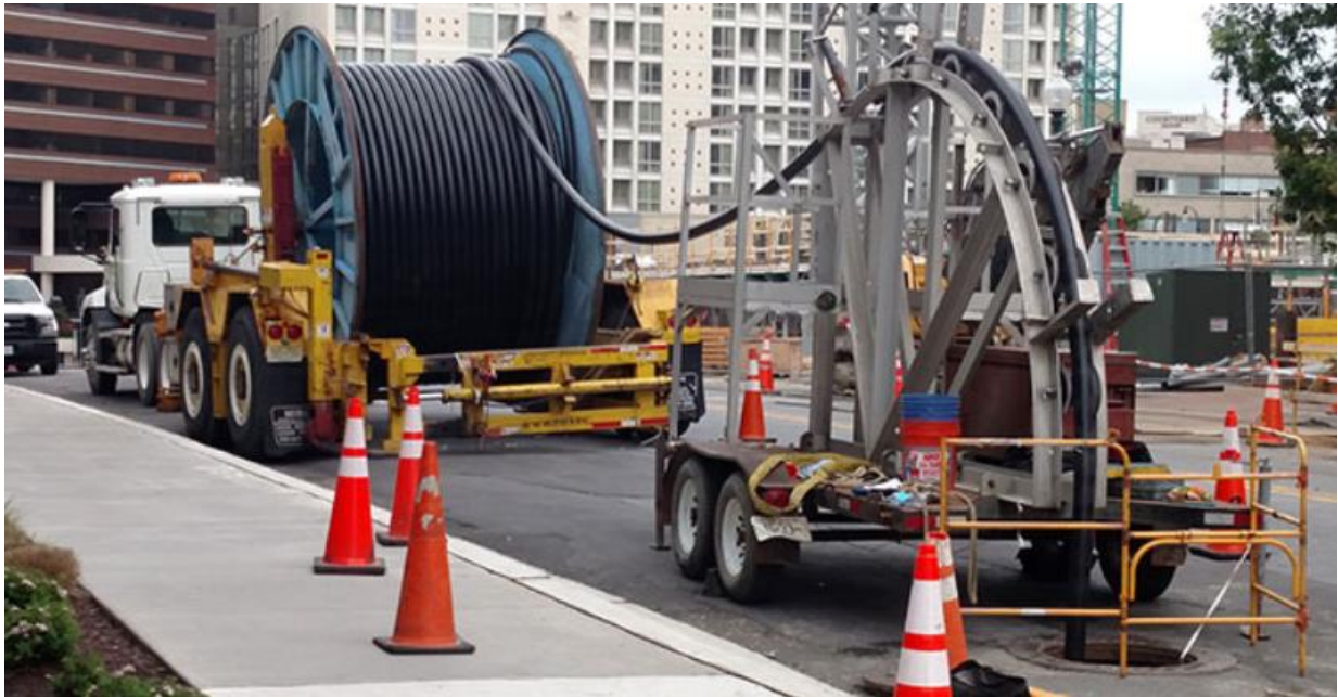
Figure 2-9 – XLPE Cable Installation
