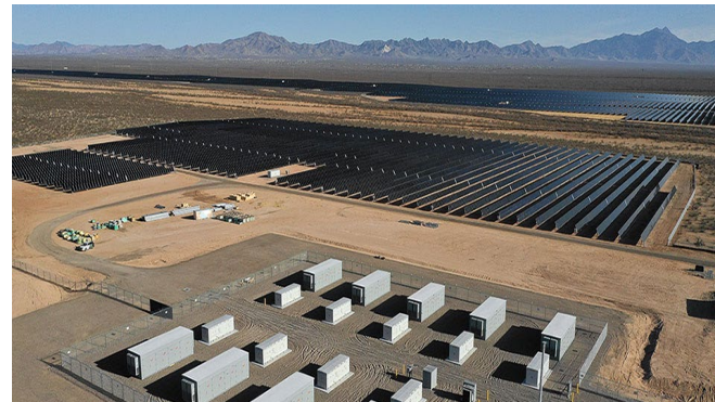
Wilmot Energy Center Tucson, Arizona 100 MW Solar and 30 MW Energy Storage
