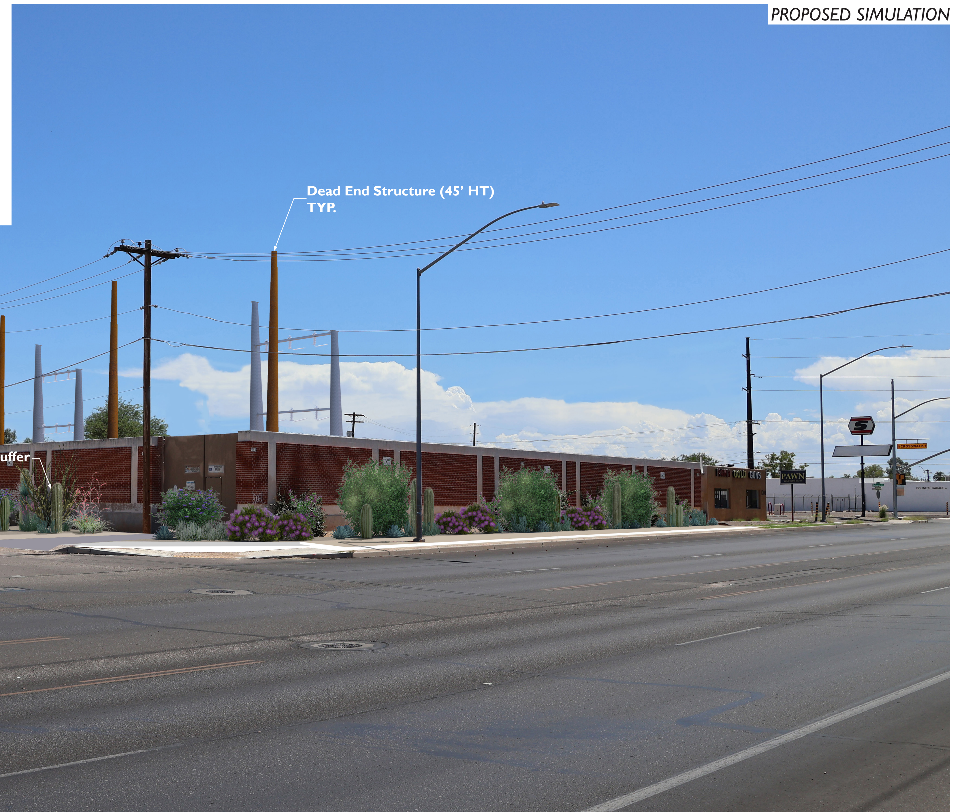
VIEW FROM WEST SIDE OF ALVERNON WAY AT THE NORTHWEST CORNER OF ALVERNON WAY AND MABEL STREET LOOKING SOUTHEAST TOWARDS THE SUBSTATION
