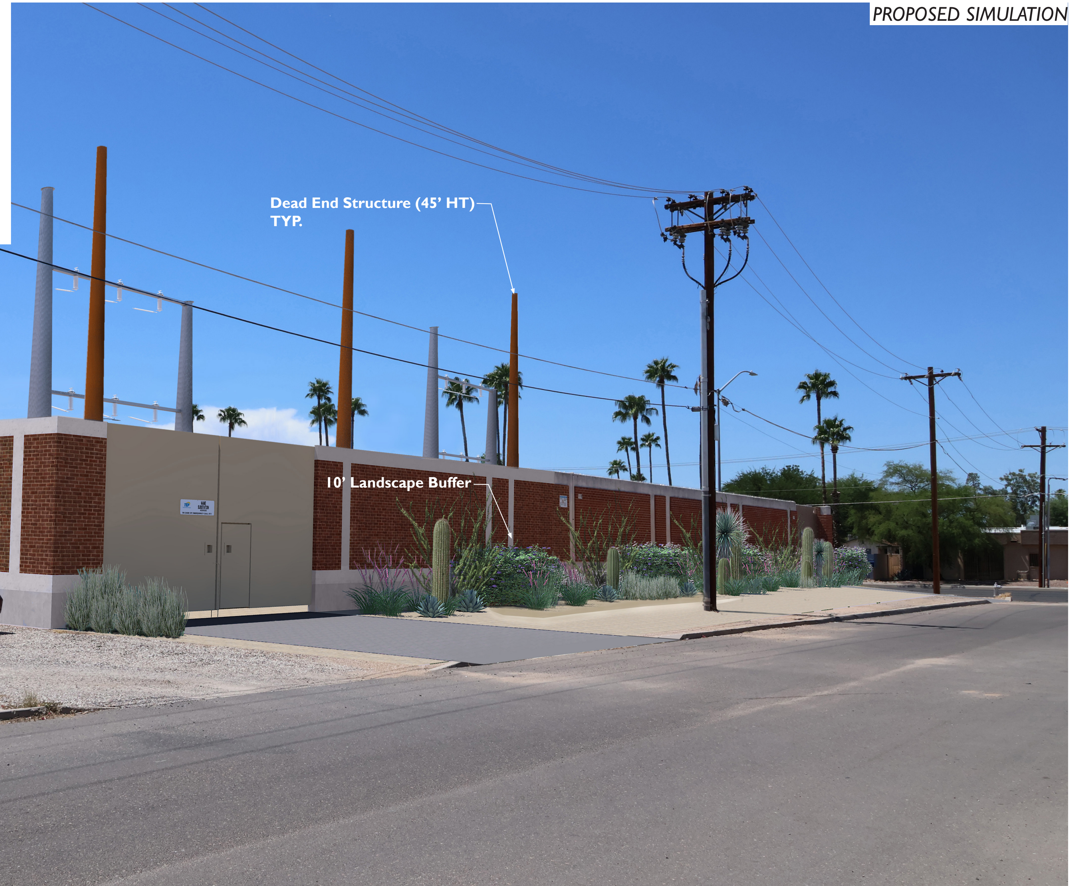
VIEW FROM MABEL STREET IN FRONT OF 3922/3924 E. MABEL ST. (DUPLEX) LOOKING SOUTHWEST TOWARDS THE SUBSTATION
