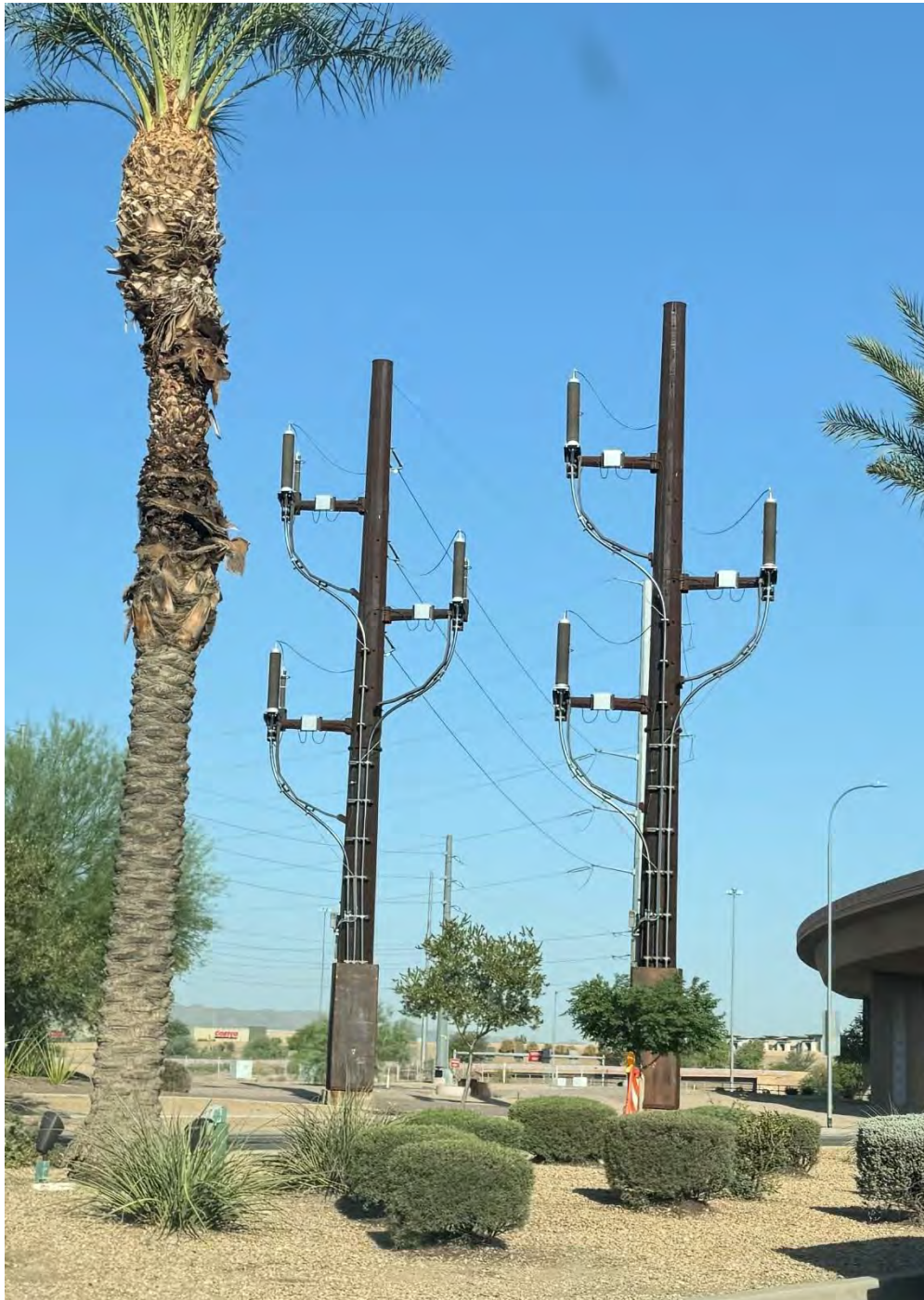
Photo 1. Example of a Steel Riser Pole (necessary if the 138 kV transmission line is undergrounded at the intersection.)
