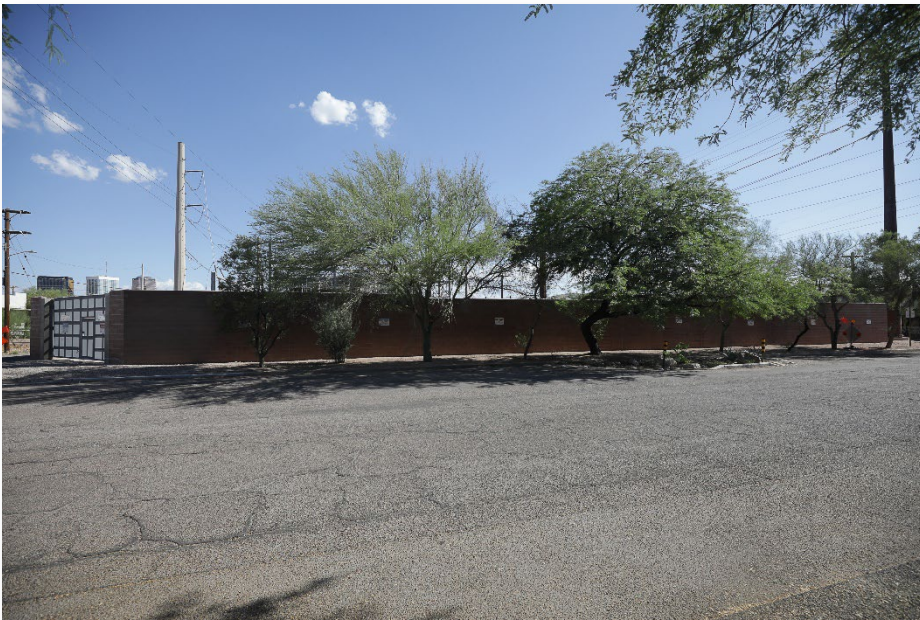
Tucson Substation, an existing GIS and Air Insulated Substation.
