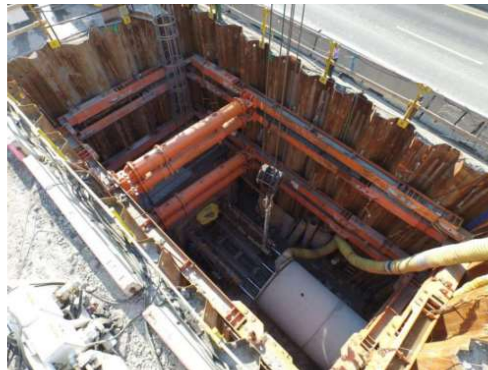
Jack-and-Bore Sending/receiving pit
