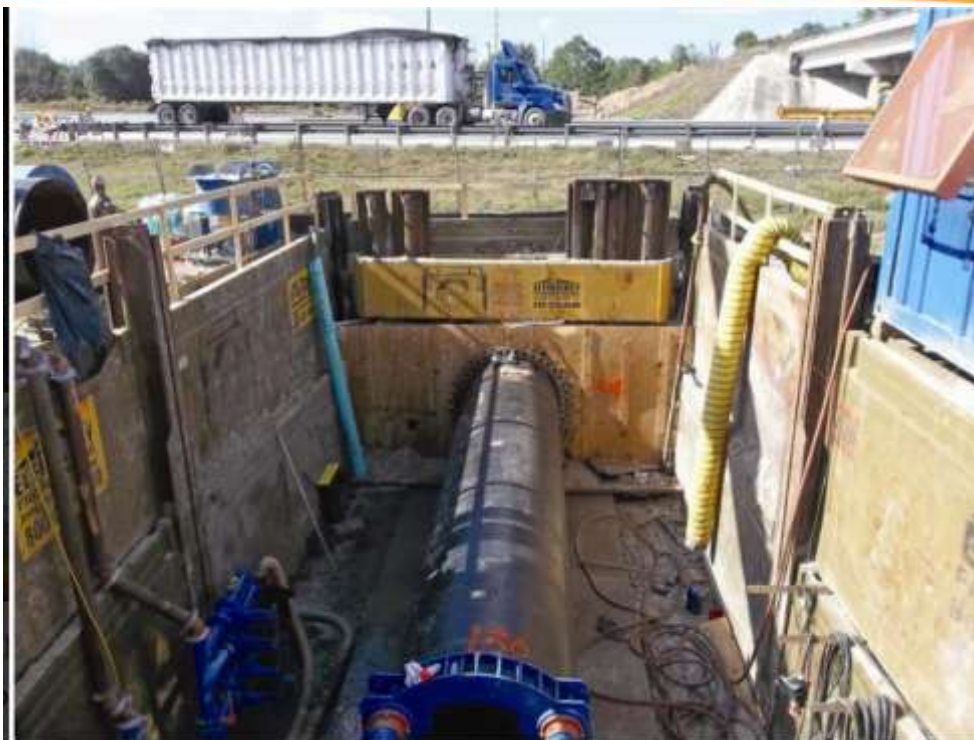
Jack-and-Bore Sending/receiving pit
