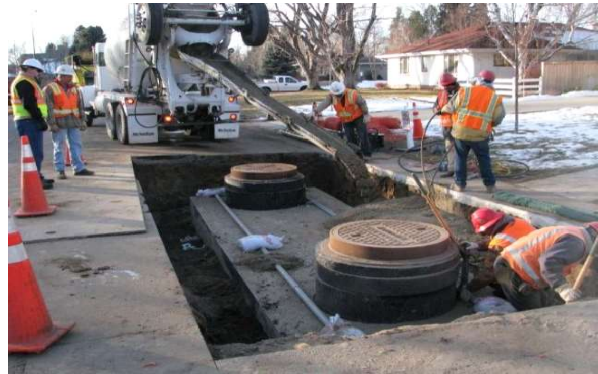
Typical HV Electric Vault Backfill
