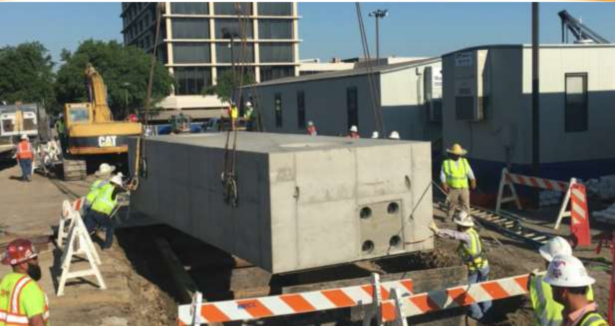
Typical HV Electric Vault Placement
