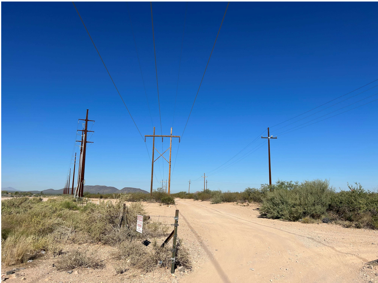
Figure 5. Field Visit (Existing Utility Corridor)
