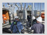
Converts electric voltage for long-distance transmission or for local customer use.
