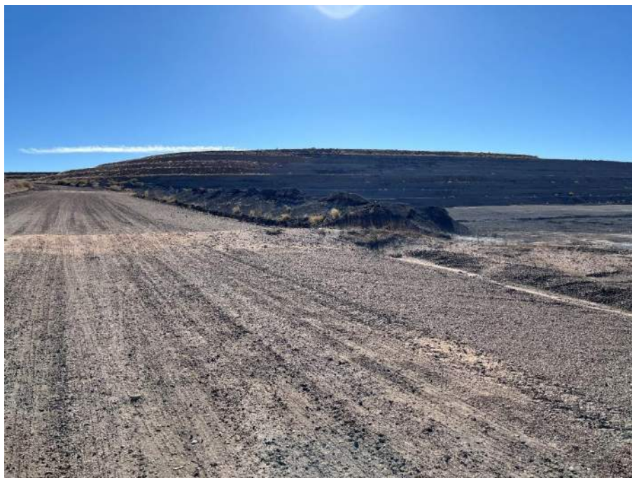
Photo 6 Water bars along perimeter haul road, directing stormwater onto Active Fill Area; facing east
