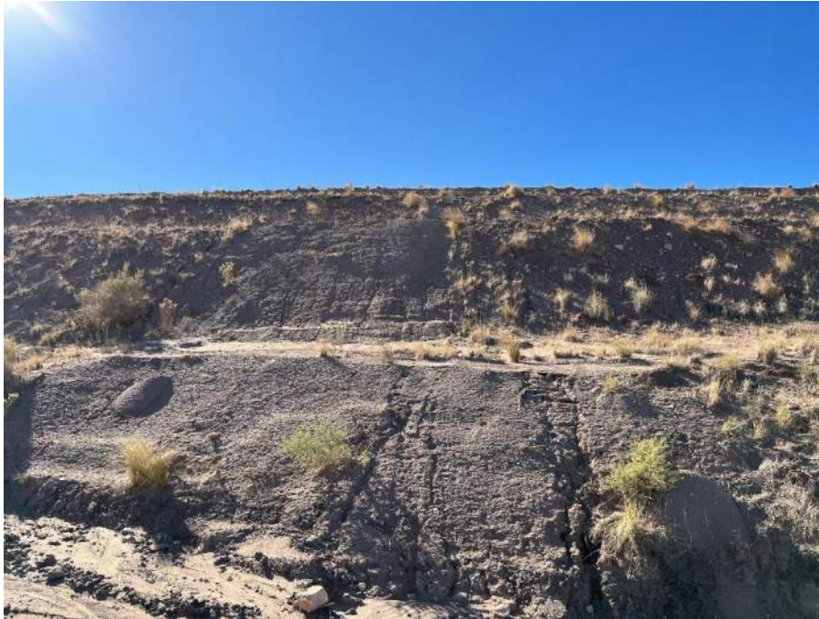
Photo 7 Repaired erosion gully on north side of Inactive Fill Area; facing south
