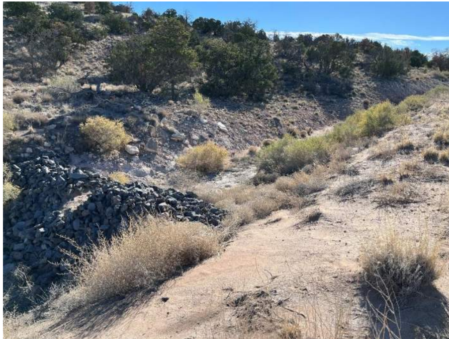
Photo 3 Rock check dam in the north perimeter drainage ditch; facing southwest
