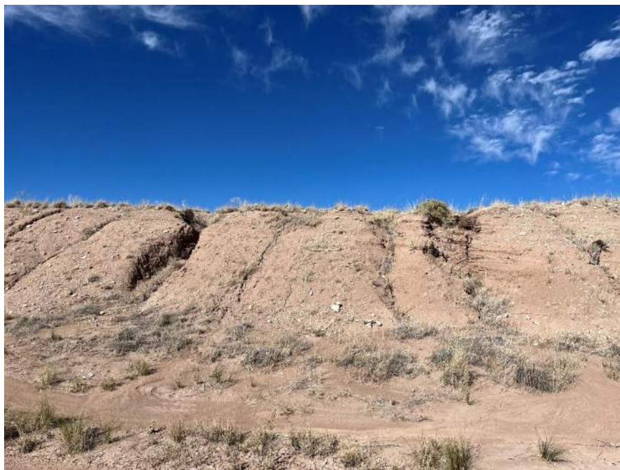
Photo 16 Deep erosion gullies on the slope; facing north
