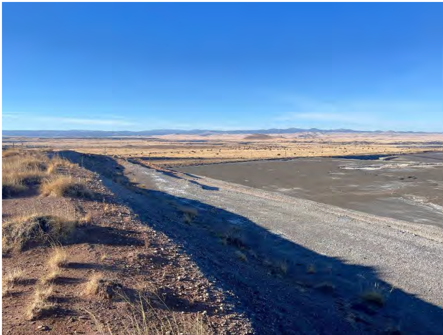
Photo 58 Typical condition of benches and side slopes along west face of Inactive Fill Area; facing southwest
