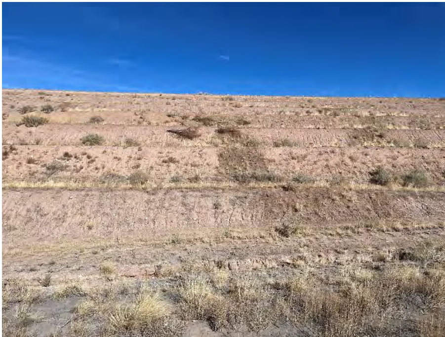
Photo 22 Typical conditions along south slope of Inactive Fill Area; facing north
