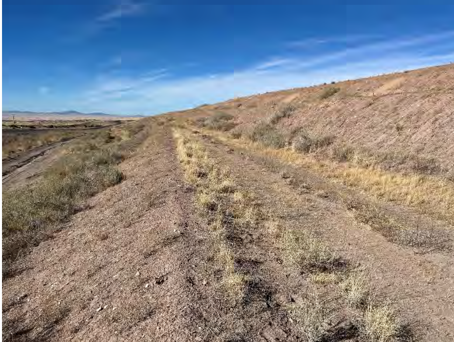
Photo 17 Typical conditions of bench along south slope of Inactive Fill Area; facing west
