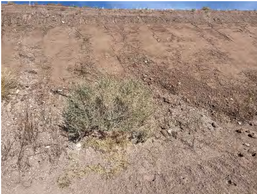
Photo 48 Repaired erosion on downhill side of bench; facing northeast
