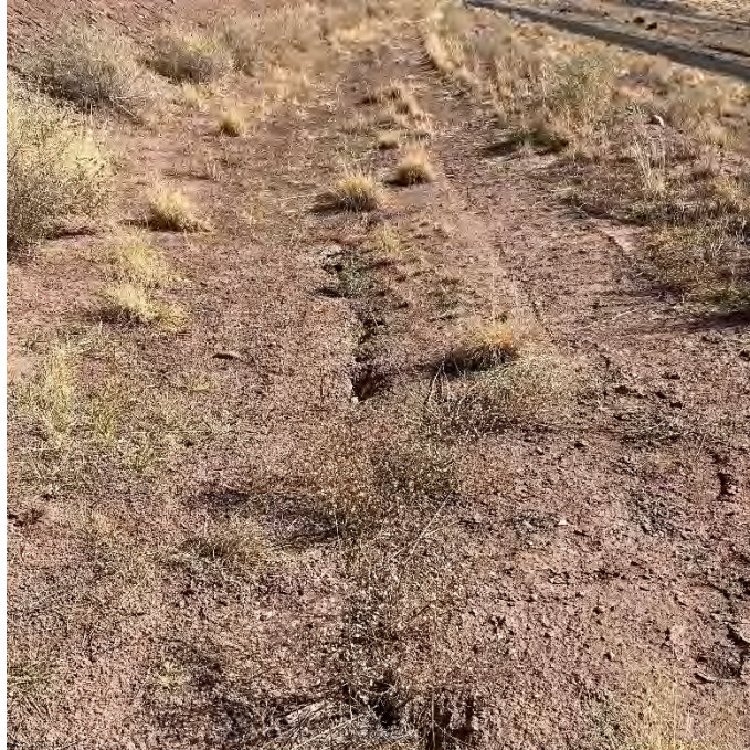
Photo 39 Cracks on the second bench from top; facing east
