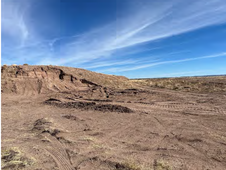
Photo 57 Topsoil stockpile in western end of Inactive Fill Area; facing northeast
