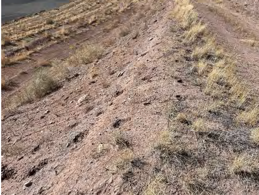
Photo 51 Animal foraging holes on side slope; facing southwest
