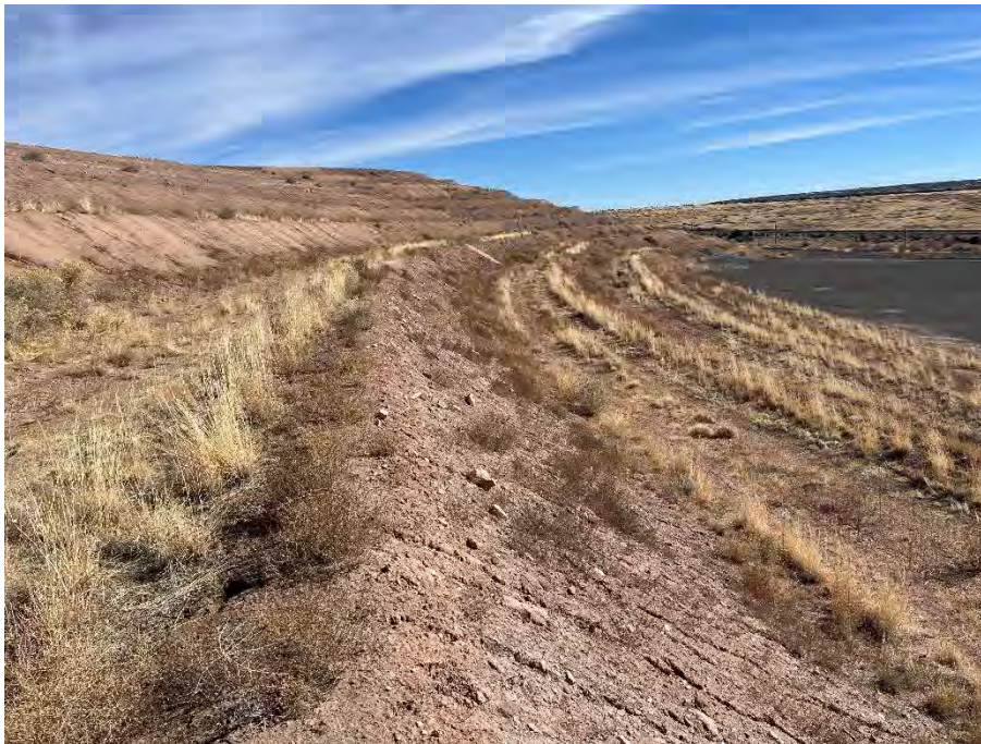
Photo 50 View of south side of Inactive Fill Area, showing soil cover and benches; facing southeast
