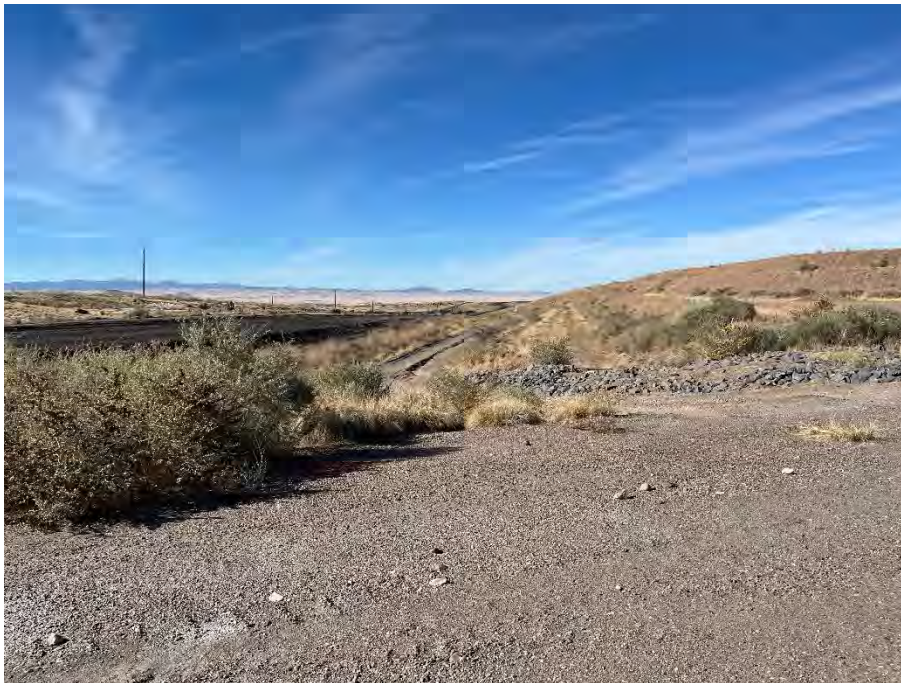
Photo 16 Side slopes and south drainage channel at the southeast corner of the landfill; facing west
