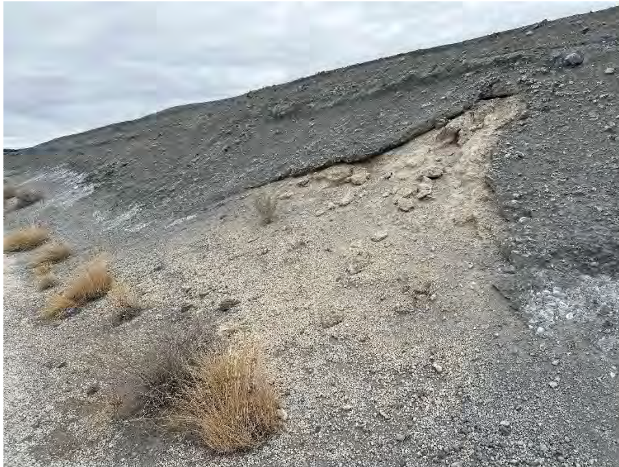
Photo 57 Isolated sloughing on downhill side of benches (light-colored fly ash exposed beneath cover layer of bottom ash)
