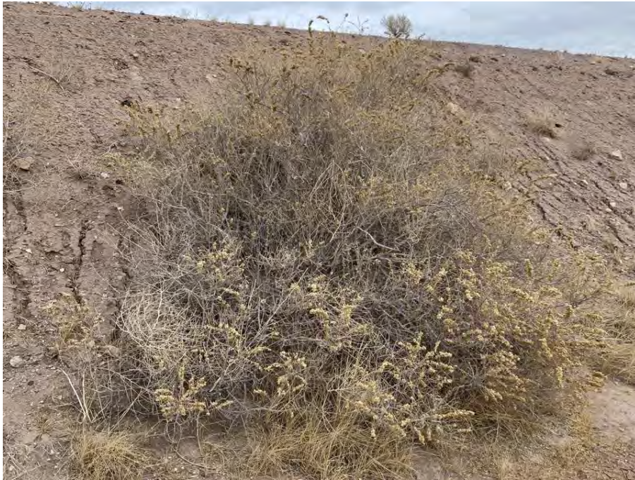
Photo 33 Woody vegetation present at toe of side slope
