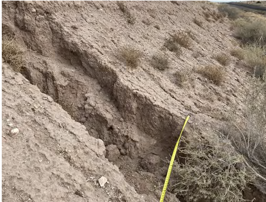
Photo 39 Closeup and scale of deep erosion gully on downhill side of bench
