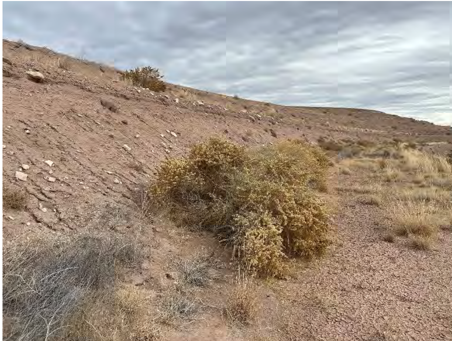
Photo 53 Woody vegetation on toe of side slope
