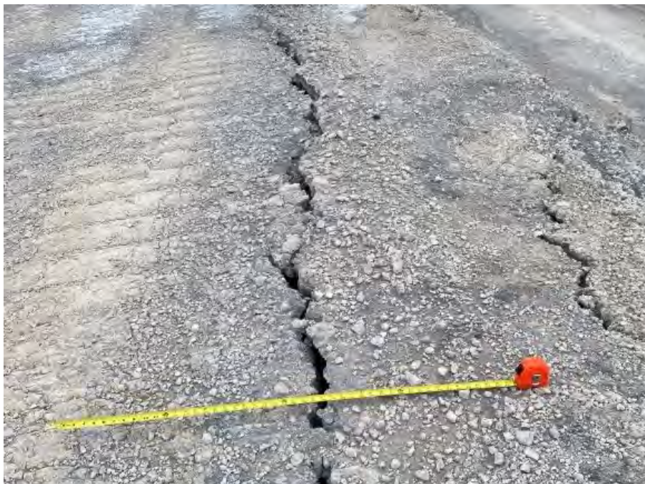
Photo 58 Tension cracking along crest of western slope in Inactive Fill Area
