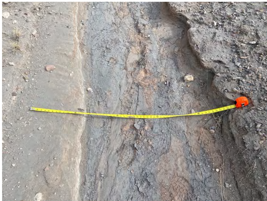
Photo 36 Typical width of incised/ eroded drainage channel at toe of south embankment
