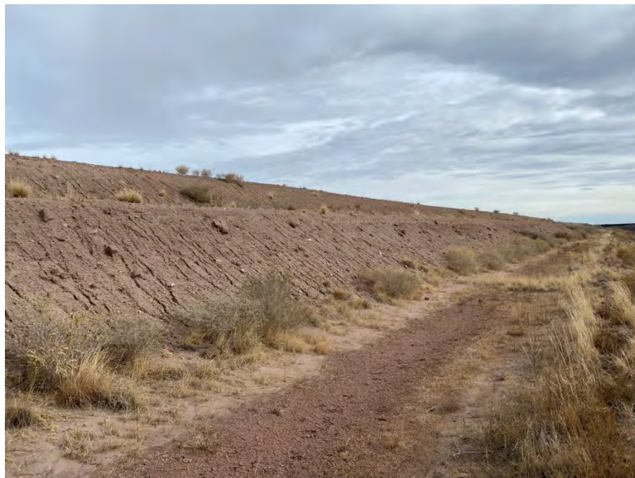
Photo 38 Pooling area between lateral confining berms on bench
