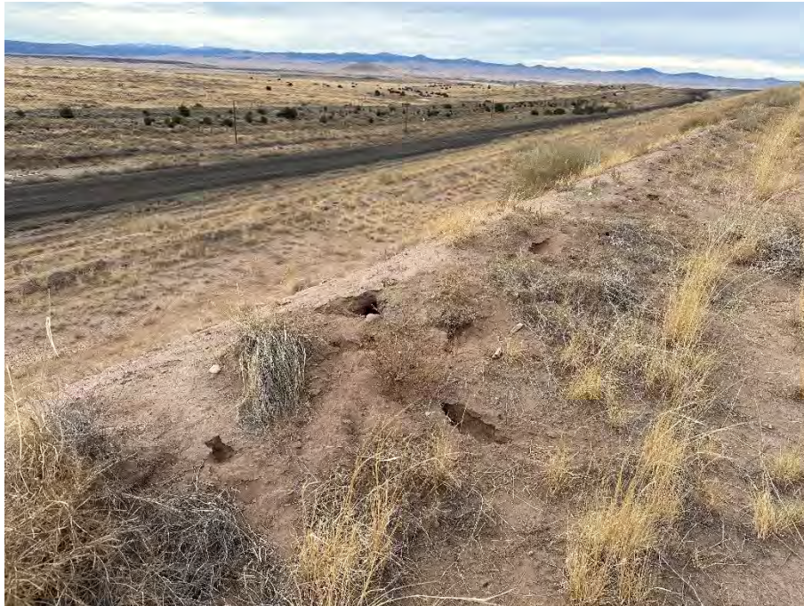
Photo 35 Animal burrows present on outer edge of bench
