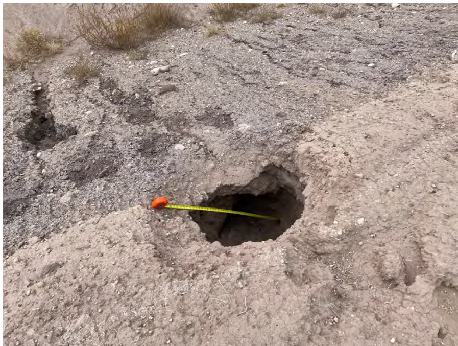
Photo 48 Small-to-moderate sized hole or cave-in at crest of berm
