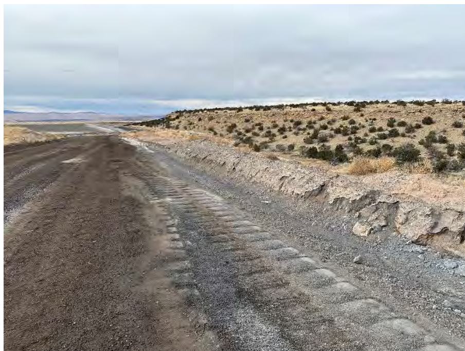
Photo 10 Typical condition of perimeter road and roadside berm, directing flow west
