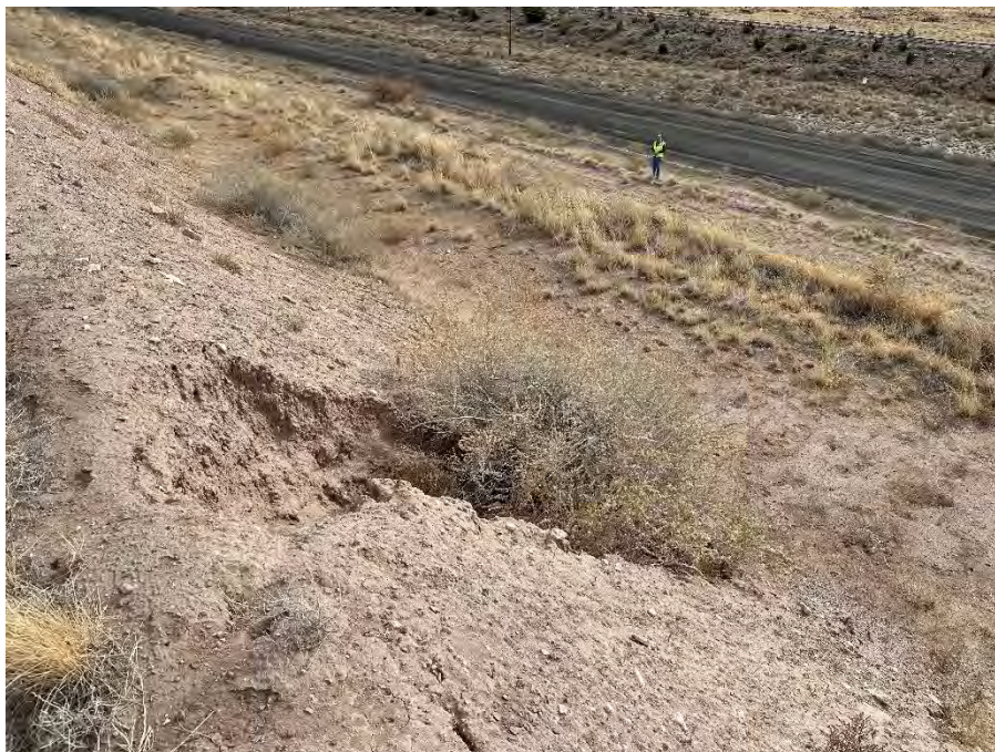
Photo 40 Deep erosion gully on downhill side of bench
