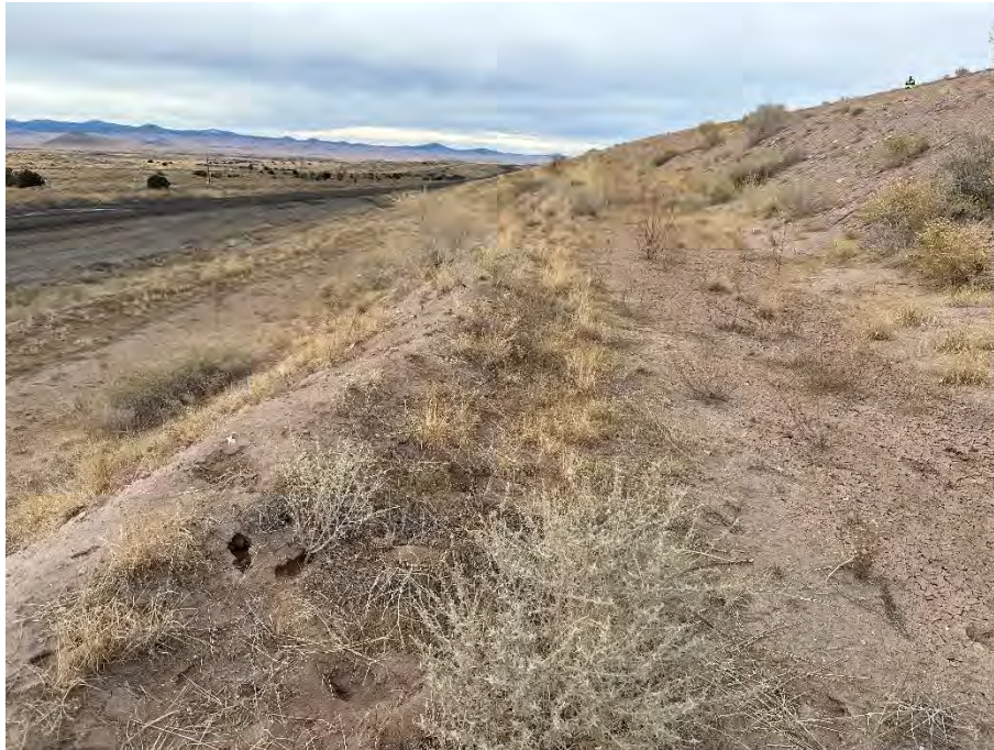
Photo 25 Animal burrows present along elevated lip on outer edge of bench
