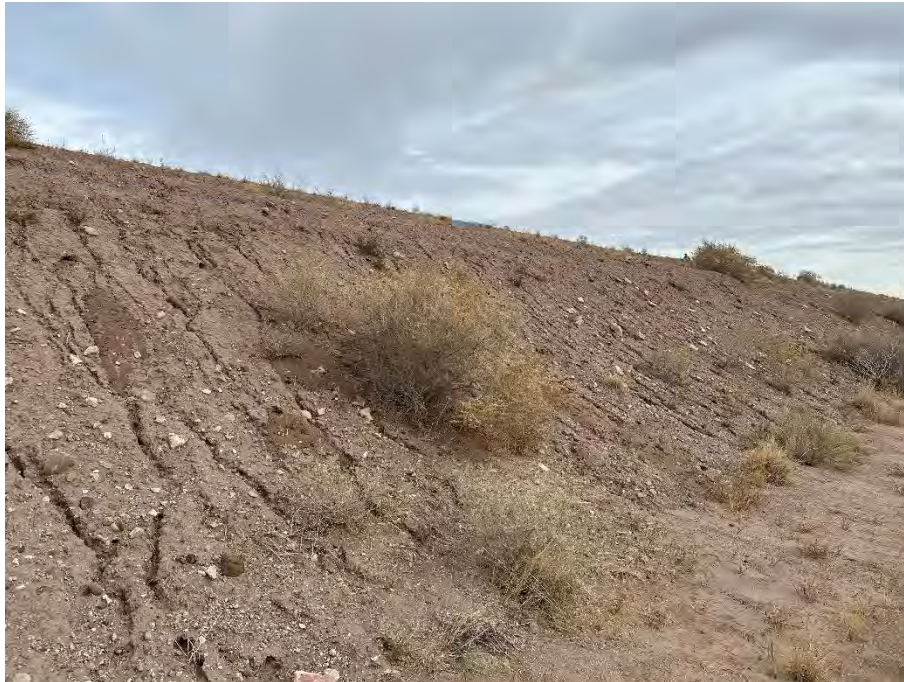
Photo 37 Typical erosion rills and vegetation along benches
