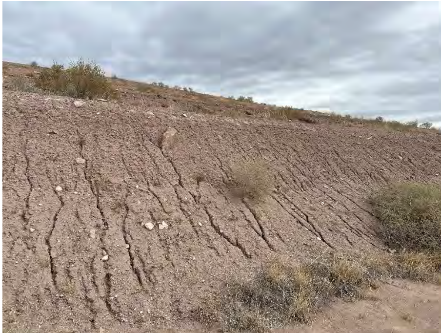
Photo 47 Typical erosion rills on downhill side of bench
