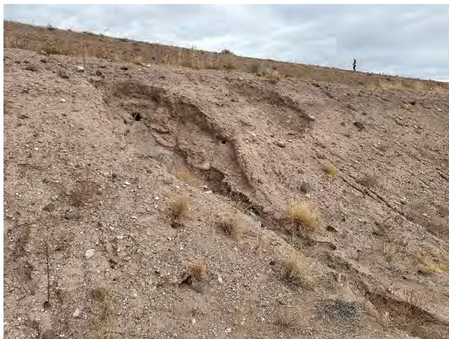
Photo 52 Erosion washout on downhill side of bench
