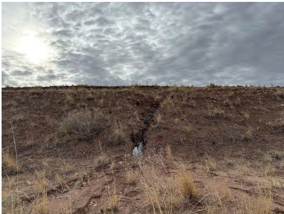
Photo 9 Erosion gully on north side of Inactive Fill Area
