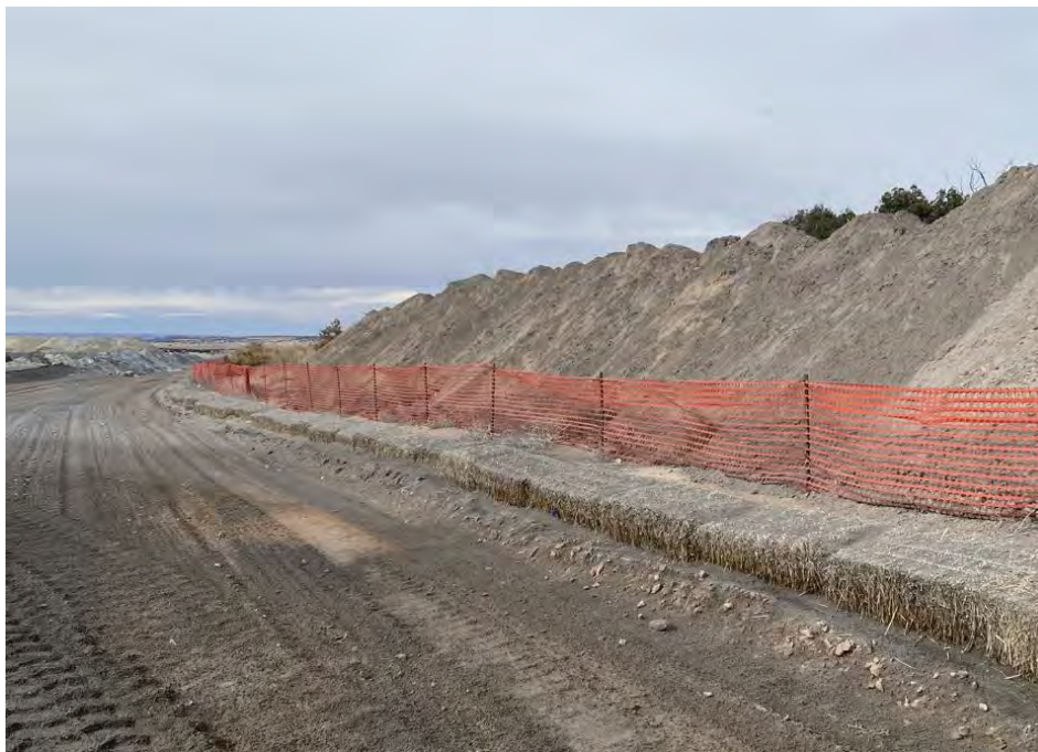
Photo 4 Erosion and sediment controls (e.g., orange construction fence and hay bales) along perimeter road
