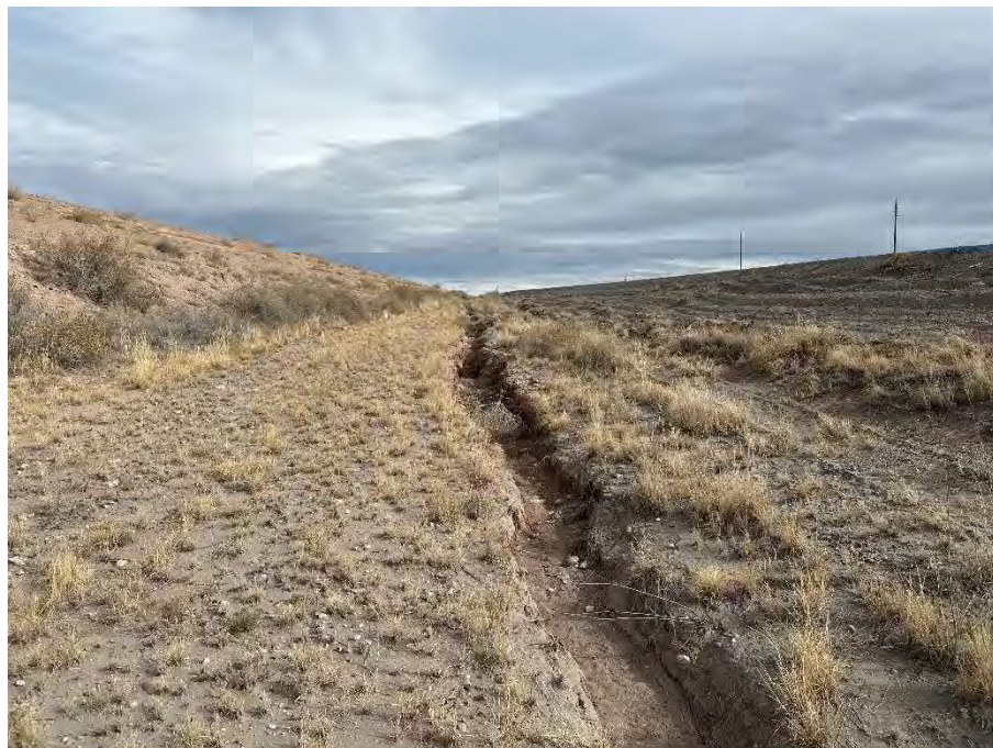
Photo 26 Incised/ eroded drainage channel at toe of south embankment and adjacent Ash Haul Road
