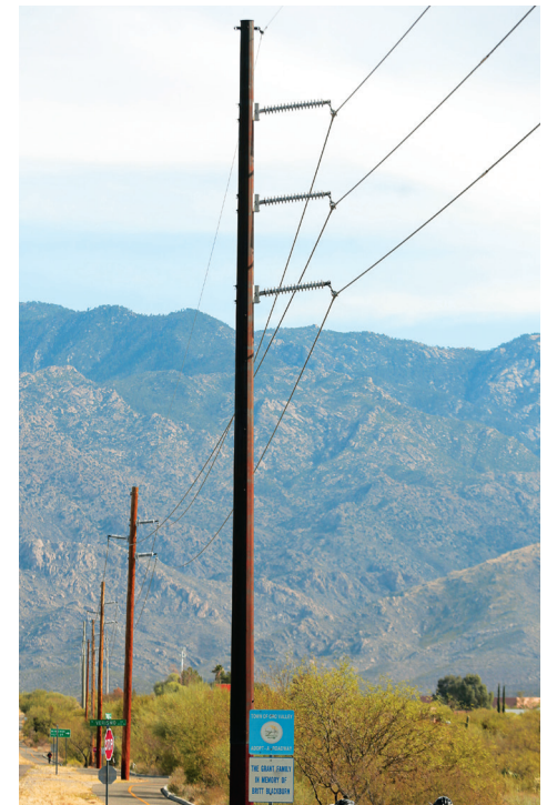
A typical weathering steel monopole supporting a 138 kilovolt transmission line.
