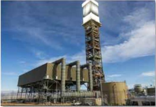
Ivanpah Solar Receiver and Condensers
