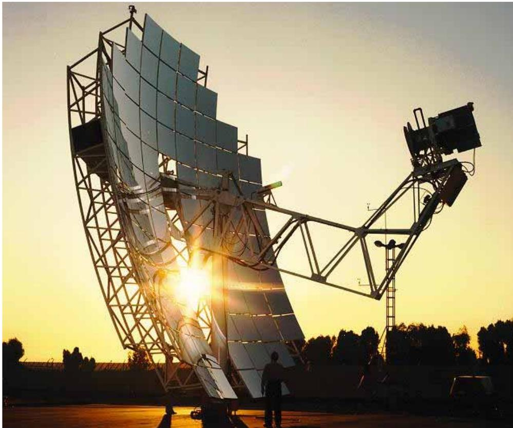
A generator is connected to the solar Stirling Engine, and waste heat from the engine is transferred to the ambient air via a radiator system. The gas is cooled by a radiator system and is continually recycled within the engine during the power cycle. The conversion process does not consume water, as is required by most thermal-powered generating systems.
