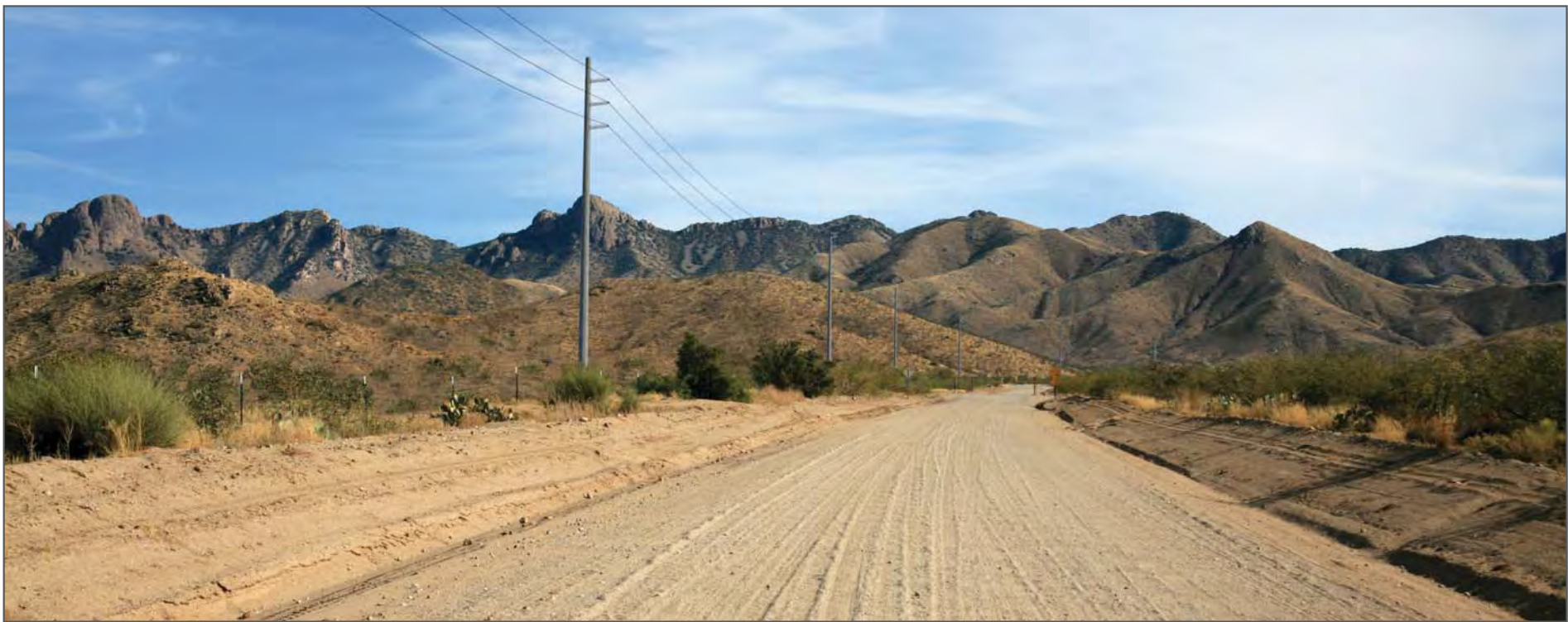
Simulated Condition – Proposed 138kV galvanized steel single-circuit transmission lines and water pipeline with shared access road
