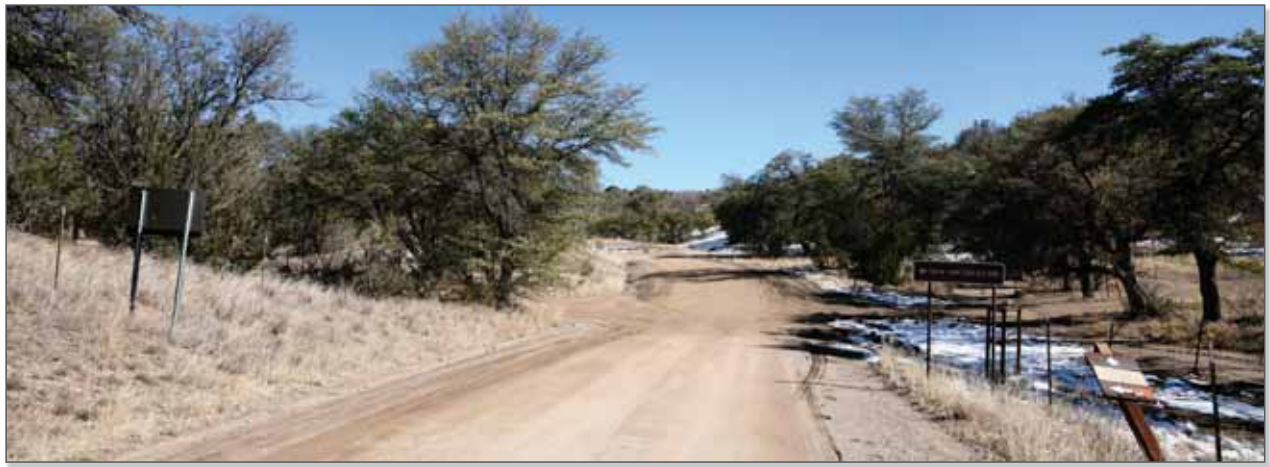
Existing Condition – Box Canyon Road within the Santa Rita Mountains
