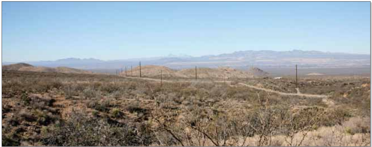
Simulated Condition – Proposed 138kV corten steel single-circuit transmission line and water pipeline with shared access road
