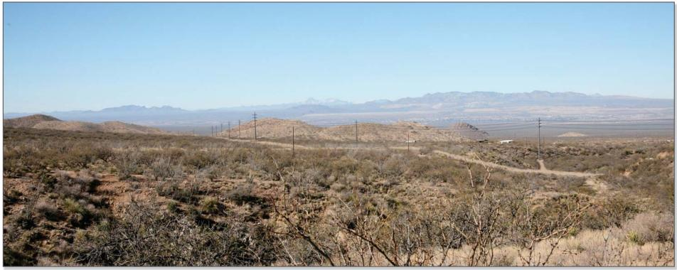
Simulated Condition - Proposed 138kV galvanized steel double-circuit transmission line and water pipeline with shared access road
