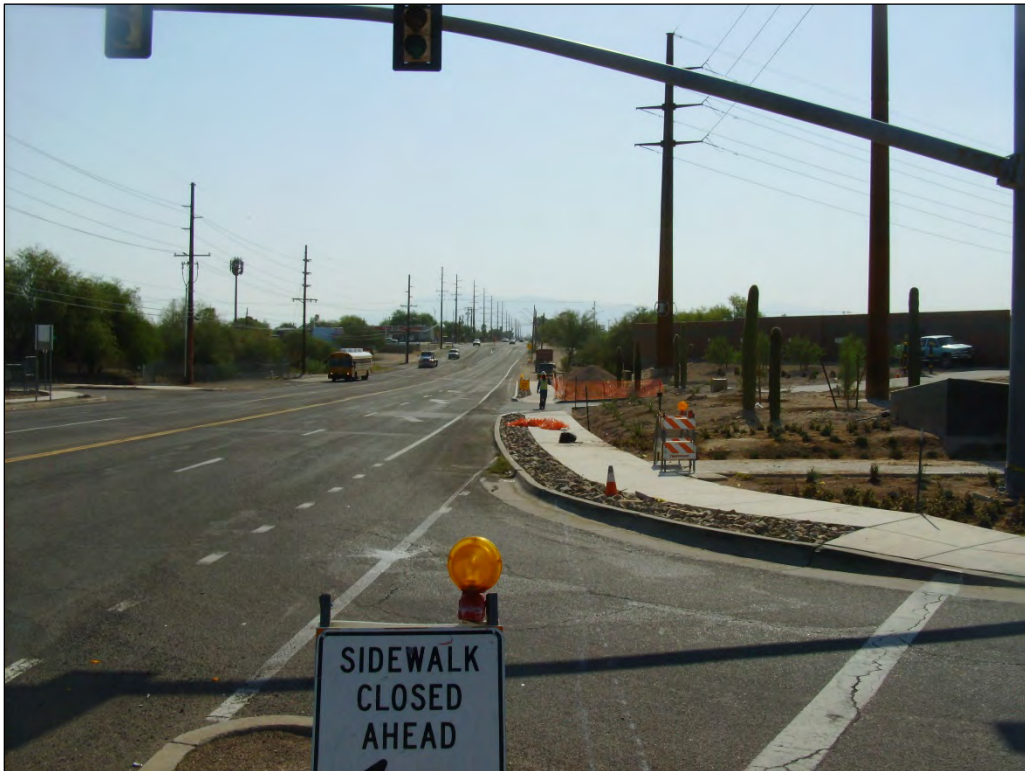
Photo 2. Alternative 2 and 5 corridor, view to west from 36th and Kino.
