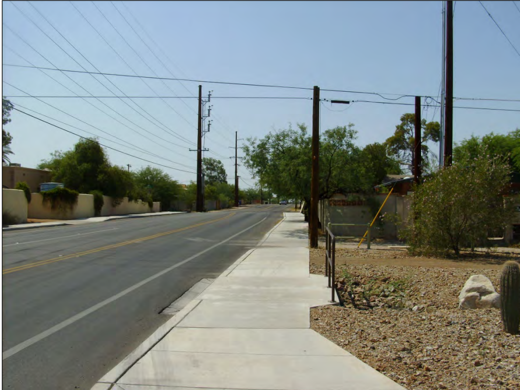
Photo 10. Alternative B corridor, view to south from Grant and Park.
