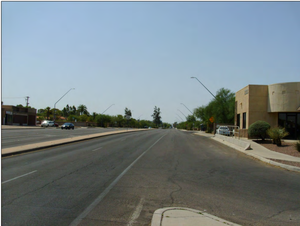
Photo 12. Alternative D corridor, view to south from Grant and Campbell.
