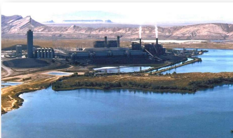
Picture 5 - Four Corners Power Plant
