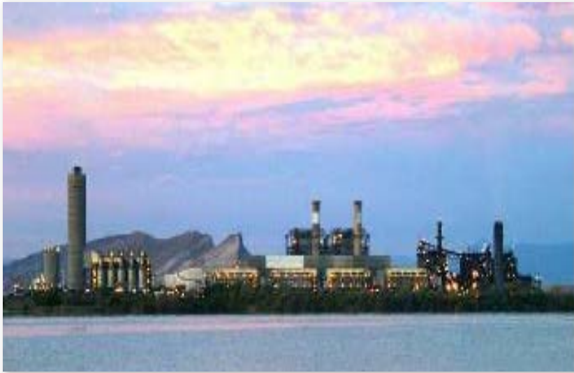
Picture 22 - Four Corners Power Plant
