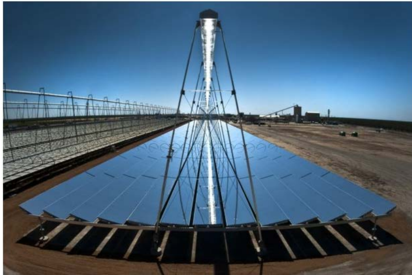
Areva Solar – Sundt Generating Station
