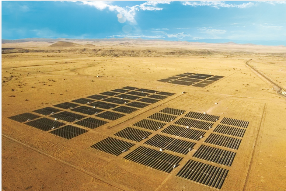
Picture 10 - Springerville Solar
