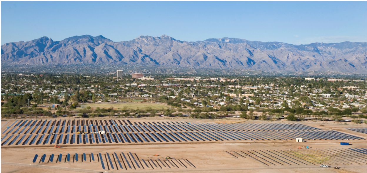
Picture 20 – Davis Monthan Air Force Base Distributed Generation Project
