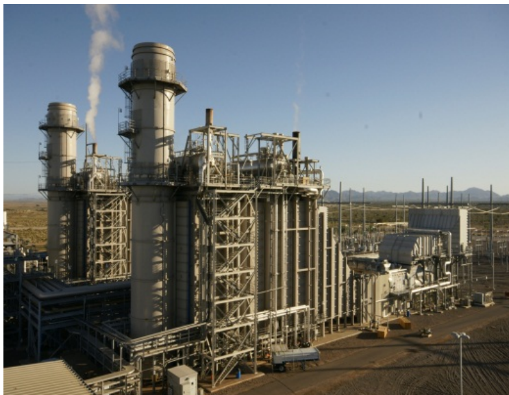
Picture 27 – Gila River Power Station
