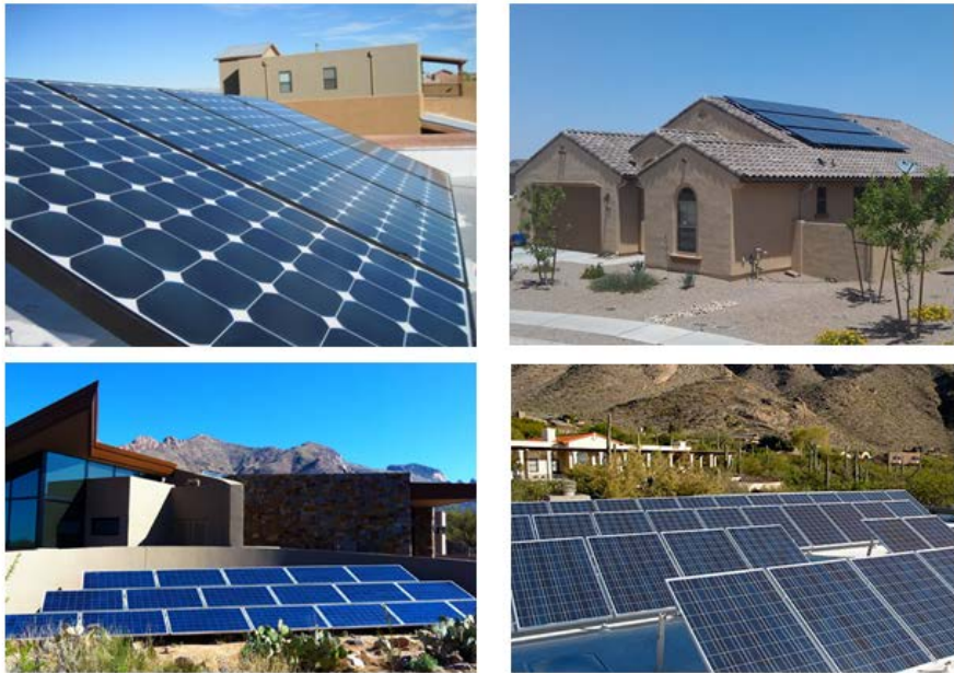
Typical residential distributed photovoltaic (PV) systems
