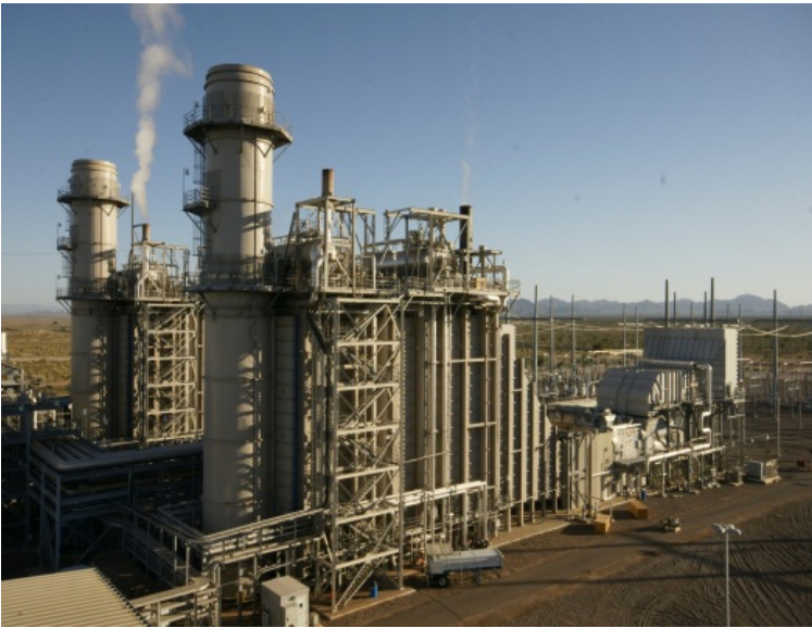
Picture 21 – Gila River Power Station
