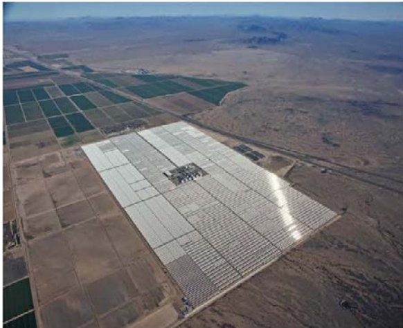
Aerial View of Solana Solar Field
